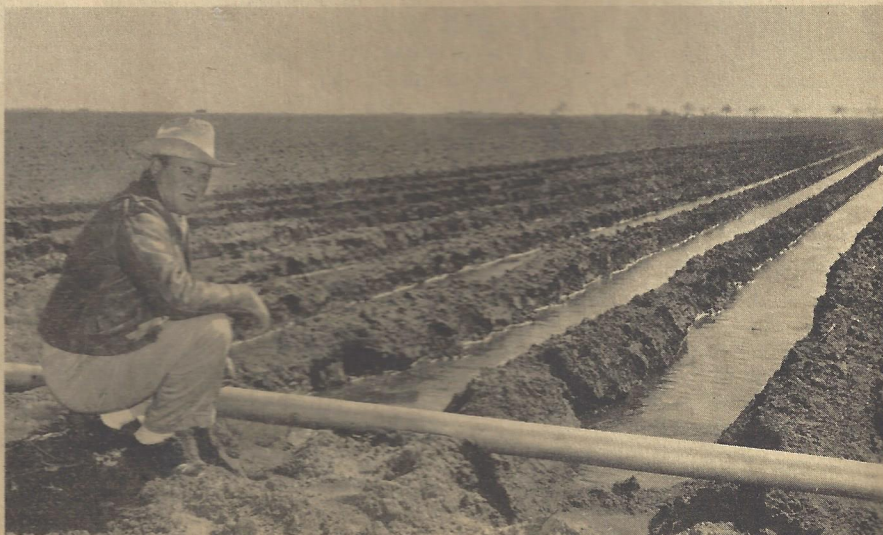
Gated pipe delivers water to parts of Schwab's acreage level enough for flooding. Here he observes the movement of water across a field.
