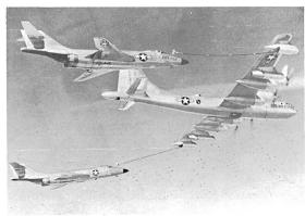
The KB-50, tanker version of the B-50 Superbomber, differs very little from the B-29/KB-29 aircraft from which it evolved. It can be identified by its considerably taller and larger vertical stabilizer; larger engine nacelles, each extending aft of the wing; and the slightly modified wing trailing edge.
